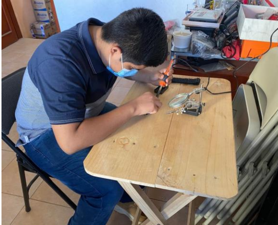
Figure A.1. Soldering gearmotor cables. Own photography.
